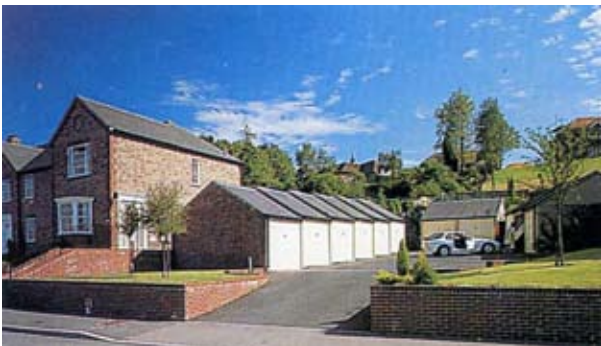
Gable end cladding in brick co-ordinates these garages with the adjacent house development. Garages are stepped to accommodate the site levels.
