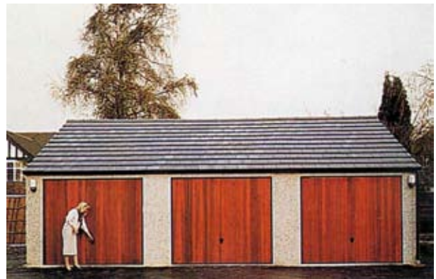
Heritage 9 garages with Marley Modern roof tiles, Marley dry ridge and dry verge, cedar vertically boarded doors and Whitespar natural stone granule wall finish.
